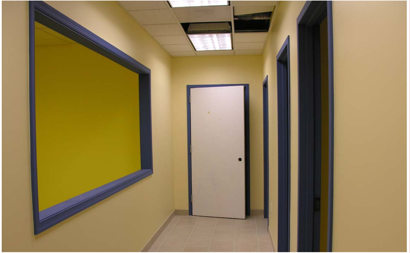
2ND STORY OFFICE SPACE
